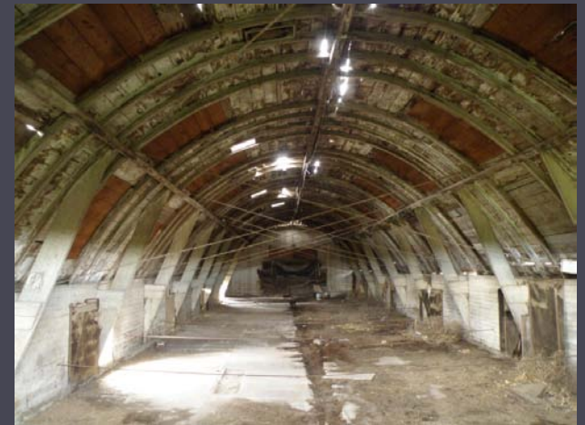
Hog barn converted to grain storage
