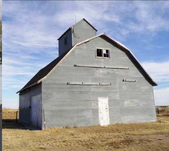
Barn converted to elevator
