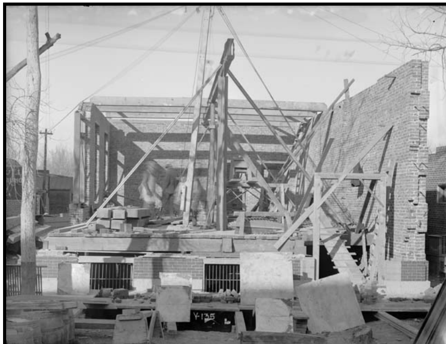
Telephone Building under construction, Colorado Springs (1897)
