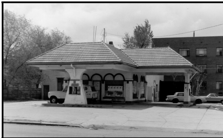
Double-canopy station in Denver
