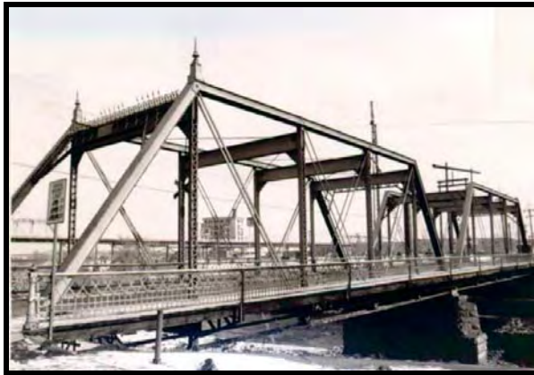
Pratt Truss, Denver
