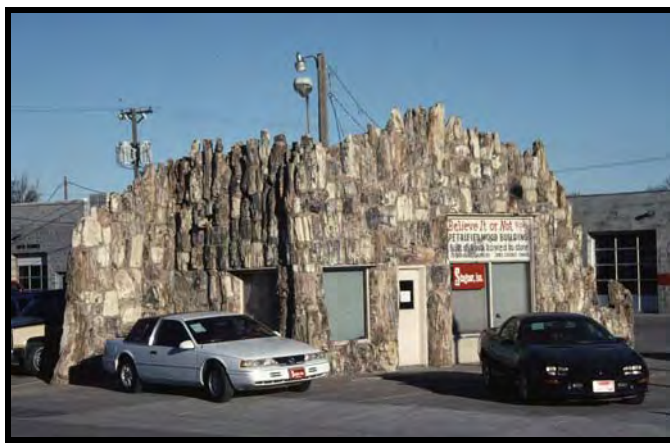
Lamar gas station made of petrified wood
