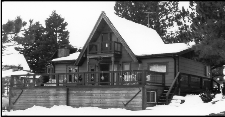
Though not a true A-Frame, this house in Louviers combines the basic form with gable-roofed side wings.
