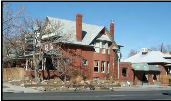
An unusual rear commercial addition in Denver
